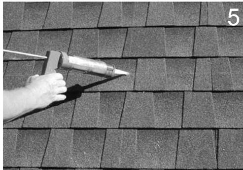
5 Clean off any saw dust, and fill hole with Sealant.
