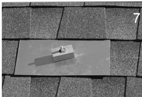
7 Insert EPDM Rubber Washer over Hanger Bolt into Block.
