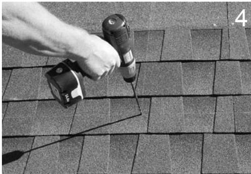
4 Using drill with 1/4" long bit, drill pilot hole into roof and rafter, taking care to drill square to the roof.
