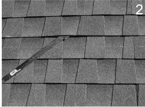
2 Lift Composition roof shingle with Roofers Bar, just above placement of Quick Mount.
