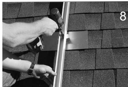
8 Using the Racking Hardware, secure the rack of your choice. Tighten to 16 foot pounds.
