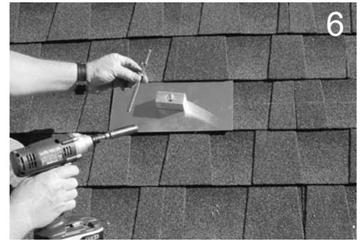
6 Slide Mount back into position. Prepare Hanger Bolt with 1 Hex Nut and 1 Sealing Washer, insert through Block into hole and drive Hanger until Block is tight.
